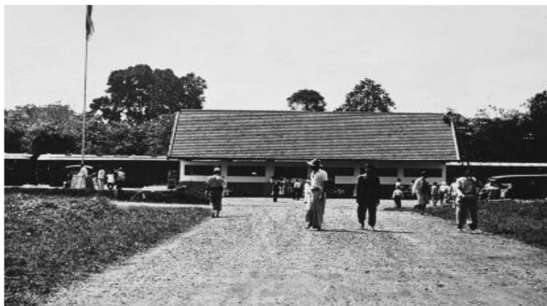
Figure 1. Lubuklinggau Railway Station, 1934
